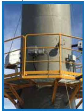
Continuously emission monitoring systems (CEMS)
