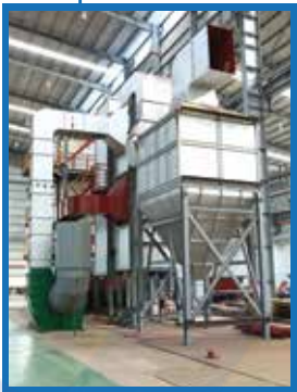
Multi-Cyclone (Pre-Filter): Filtration efficiency from 80% to 90%
