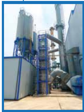
Absorption Tower : SO x absorption/reduction
